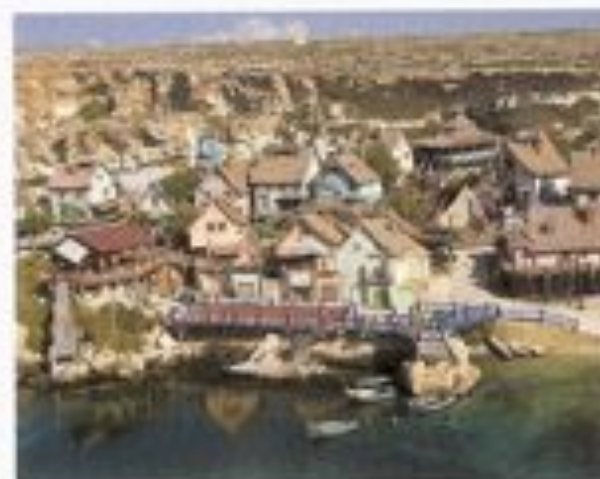
Popeye (feature) - MFS set construction for location shoot, 1980
